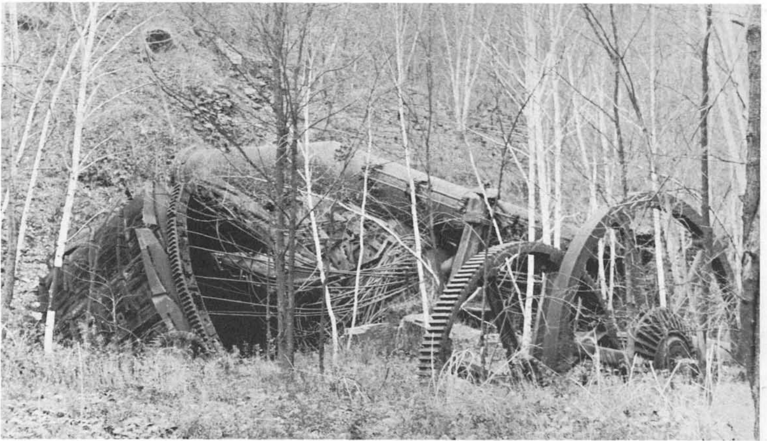
Figure 14. Burden's Great Wheel, as it lay in ruins during the period between collapse of the brick bearing pier in 1914 and final scrapping before World War II. Photograph from the L. N. Edwards Collection, Division of Mechanical & Civil Engineering, National Museum of History & Technology.
