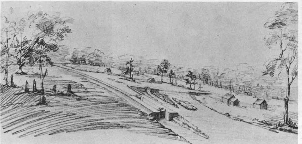
Figure 14. "Edmon's 1832" A typical lock station of the second type, with an overflow dam. Sketch by Capt. John Burrows (see page 12).
