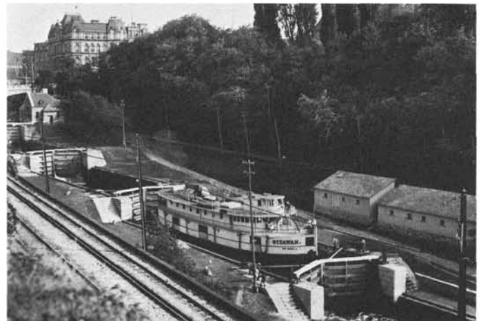
Figures 17 and 18. Steam comes to the Rideau. Left: The Kingston Mills Lock Station, c1880, with one of the lightly-constructed propeller-driven barge-tugs then coming into use. The locks here were constructed along the wall of a narrow gorge. Right: The flight of seven locks at Ottawa, the final descent of the Rideau into the Ottawa River, 1912. Ottawa Forwarding Co. Steamer, Ottawan ; Hull Electric and Canadian Pacific Railway tracks in the foreground. W. J. Topley photos.
