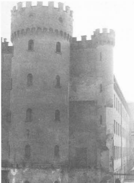
Figure 2. Cotton mill at Vaprio d'Adda, near Bergamo, second half of the nineteenth century.
