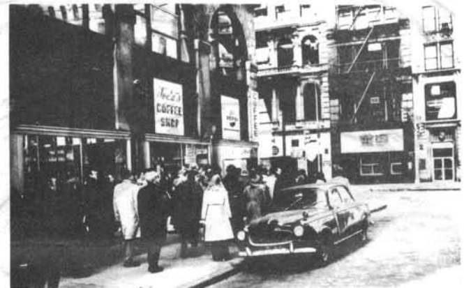
In the heart of the Cast-Iron District
