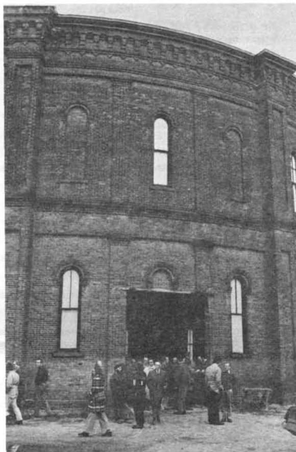
Conferees at the Troy Gas Light Company Gasholder House on the Sunday tour of the Troy Area's I A.
