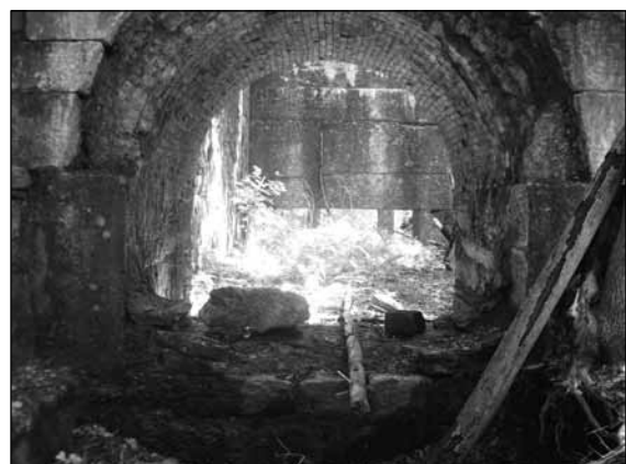
The William Stanley-designed power station was abandoned after the new generator went online upstream at Glendale. The views on this page are inside and out of the main chamber; water left here through twin passages (top) to the turbine system. The lower photo on the next page may be the base for one of the generators. (2013)
