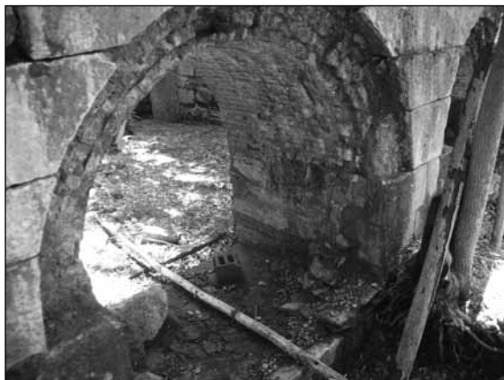
The William Stanley-designed power station was abandoned after the new generator went online upstream at Glendale. The views on this page are inside and out of the main chamber; water left here through twin passages (top) to the turbine system. The lower photo on the next page may be the base for one of the generators. (2013)
