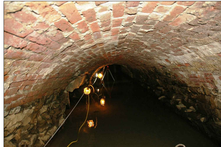
#139 STA 30 (LOOKING WEST): BRICK VAULT IS IN VERY GOOD CONDITION
