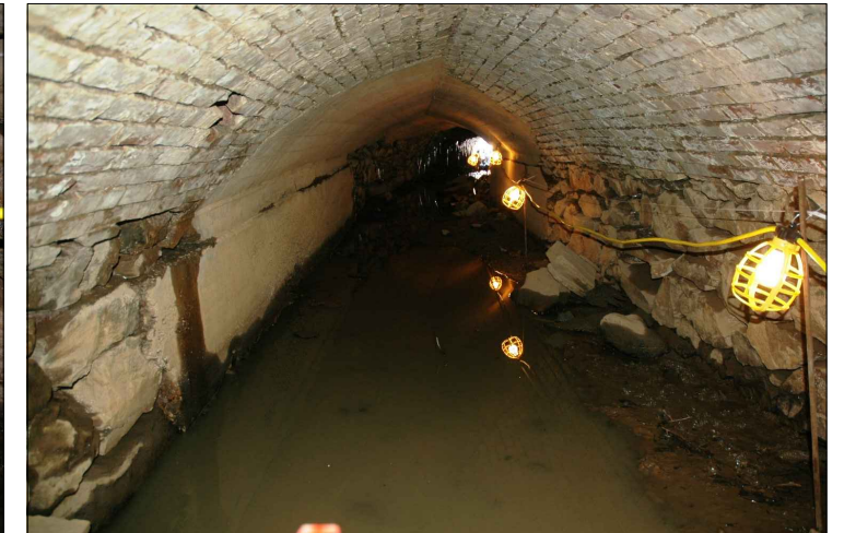
#06 STA 102 (LOOKING EAST): BRICK ARCH IS VAULTED & COMES TO A POINT
