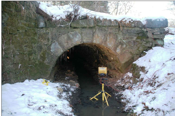
#103 STA 214: HEAD WALL, EAST SIDE OF TAILRACE
