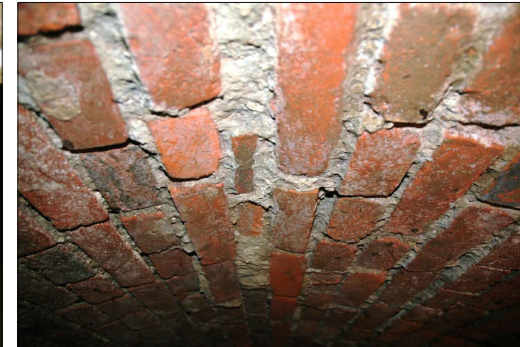
#125 STA 10: OVERHEAD BRICKS ARE IN GOOD CONDITION
