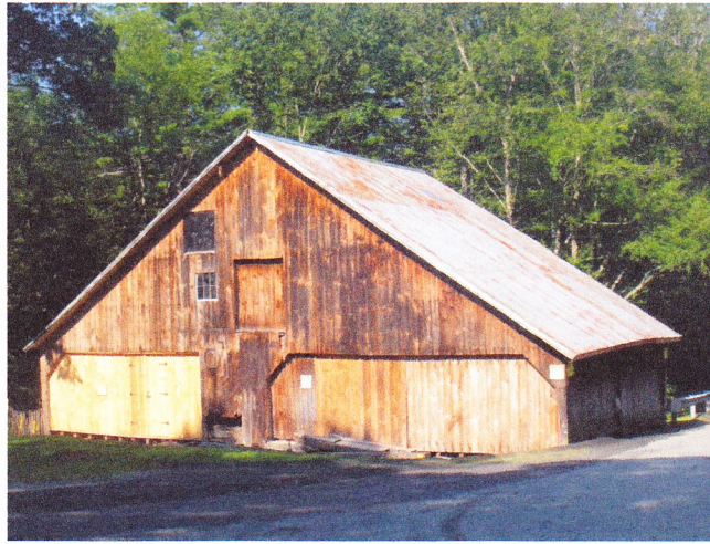
East Elevation from Old Turnpike Road, Woodstock, CT
