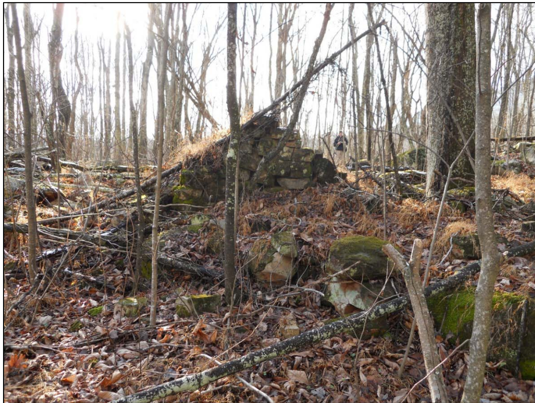
Figure 2. A portion of the foundation from the associated commissary site.
