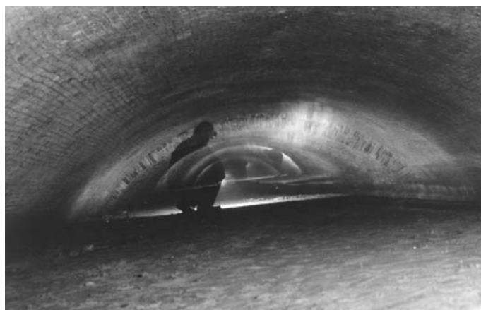
Cincinnati & Whitewater Canal Tunnel, Hamilton Co., OH.
