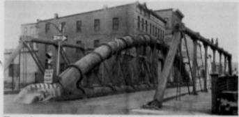
The unique span provides dual service: two traffic lanes are carried within three lines of trussing of which the two outer are conventional Pratt-type of cast and wrought iron; while the center line is a bowstring truss with top and bottom chords forming 30-inch watermains, bifurcated at the ends, carrying municipal supply. A scheme for re-erection of the remarkable structure elsewhere in the city is being examined.
