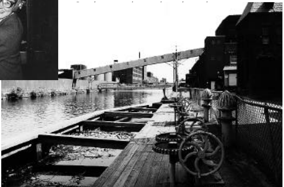
View of industrial landscape looking northeast on the second-level canal, Holyoke. Participants toured the canal system that provided waterpower to the paper and textile mills.
