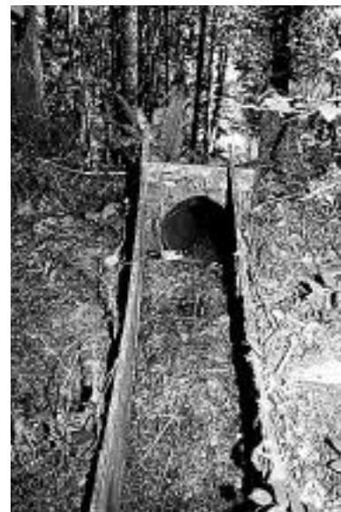
From the ditch, water was collected into a wooden headgate.
