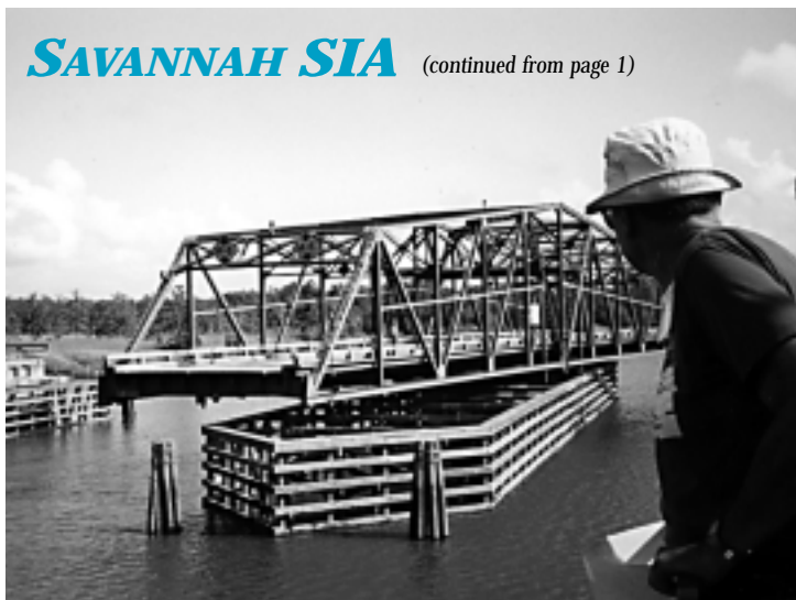
The Houlihan Bridge (1954), a swing span, was opened by special arrangement with Georgia DOT for the SIA's riverboat tour.
