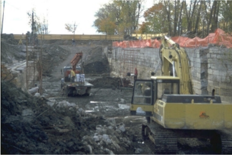
Excavation of Lock No. 5.
