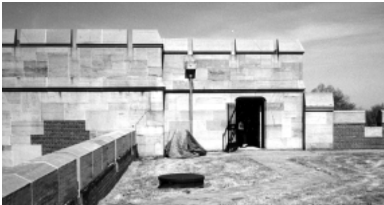
A view on the roof of the reservoir.
