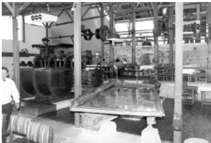
Jig, shaking table, and line shafting of a former stamp mill, now a café in Potosí.
