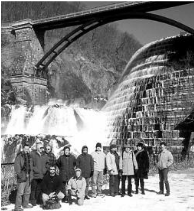
The hale and hearty take a break from the SIA winter retreat to inspect the Croton Aqueduct. Standing, l to r: Paul White, Pat Martin, Chris Andraea, Bode Morin, Carol Poh Miller, Richard Anderson, Fred Quivik, Gerry Weinstein, Louise Trotter, Rick Greenwood. Foreground: Matt Kierstead and Mary Habstritt.
