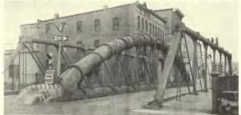
The unique span provides dual service: two traffic lanes are carried within three lines of trussing of which the two outer are conventional Pratt-type of cast and wrought iron; while the center line is a bowstring truss with top and bottom chords forming 30-inch watermains, bifurcated at the ends, carrying municipal supply. A scheme for re-erection of the remarkable structure elsewhere in the city is being examined.
