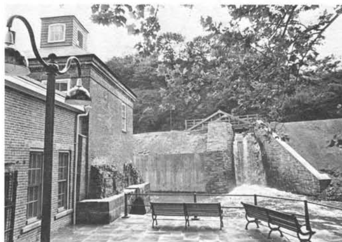
Ivanhoe wheelhouse and spillway as they appear today, restored as part of Raceway Park.
