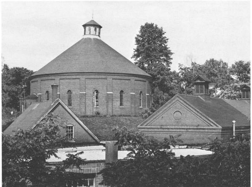
Concord (N.H.) gasholder house, believed to be the only such structure in the U.S. that survives with its iron gasholder intact. It was built in 1888 by the Concord Gas Light Co. In the foreground are the compressor (left) and purifier buildings. Gary Samson photograph.
