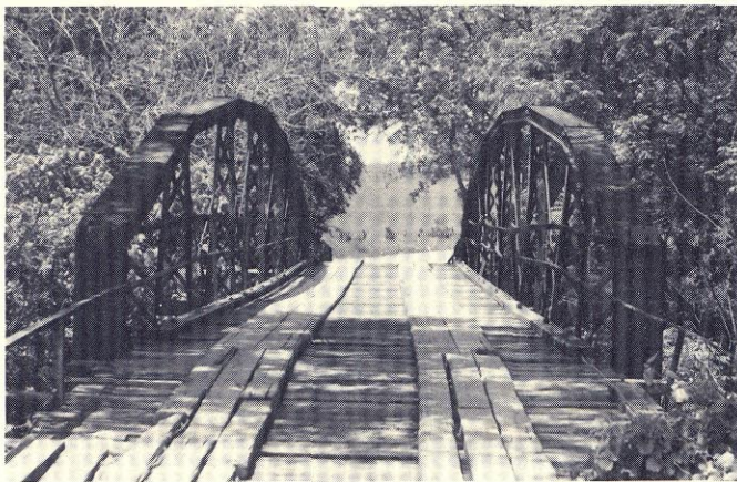
TEXAS LENTICULAR TRUSSES OUTSIDE SAN ANTONIO. All were built in the 1890s by the Berlin Iron Bridge Co. Above left: Yancey Road Bridge over Hondo Creek, Frio County. This is one of the state's two lenticular through-trusses. Above right: County Road 133 Bridge at Dodds Creek, Coryell County, revealing the characteristic double-convex-lens profile created by the top and bottom chords. Below left: County Road 173 Bridge over Plum Creek, Caldwell County. Below right: End panel of County Road 230 Bridge over Plum Creek, Caldwell County. Tex. St. Dept. of Hwys. & Trans. photographs.
