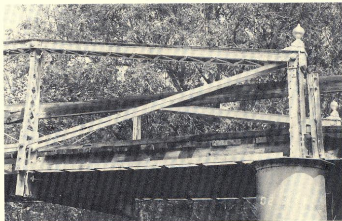
TEXAS LENTICULAR TRUSSES OUTSIDE SAN ANTONIO. All were built in the 1890s by the Berlin Iron Bridge Co. Above left: Yancey Road Bridge over Hondo Creek, Frio County. This is one of the state's two lenticular through-trusses. Above right: County Road 133 Bridge at Dodds Creek, Coryell County, revealing the characteristic double-convex-lens profile created by the top and bottom chords. Below left: County Road 173 Bridge over Plum Creek, Caldwell County. Below right: End panel of County Road 230 Bridge over Plum Creek, Caldwell County. Tex. St. Dept. of Hwys. & Trans. photographs.
