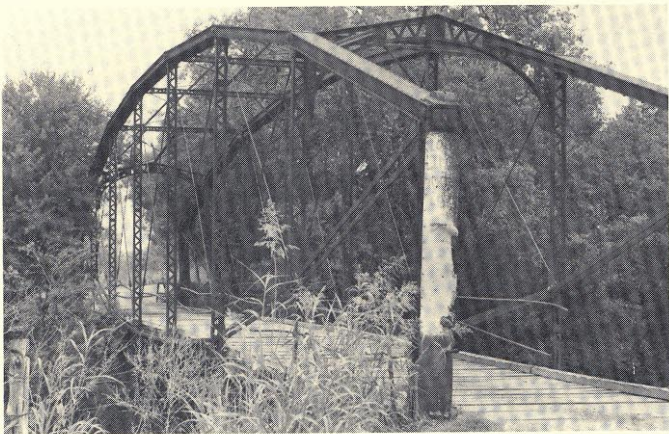
TEXAS LENTICULAR TRUSSES OUTSIDE SAN ANTONIO. All were built in the 1890s by the Berlin Iron Bridge Co. Above left: Yancey Road Bridge over Hondo Creek, Frio County. This is one of the state's two lenticular through-trusses. Above right: County Road 133 Bridge at Dodds Creek, Coryell County, revealing the characteristic double-convex-lens profile created by the top and bottom chords. Below left: County Road 173 Bridge over Plum Creek, Caldwell County. Below right: End panel of County Road 230 Bridge over Plum Creek, Caldwell County. Tex. St. Dept. of Hwys. & Trans. photographs.
