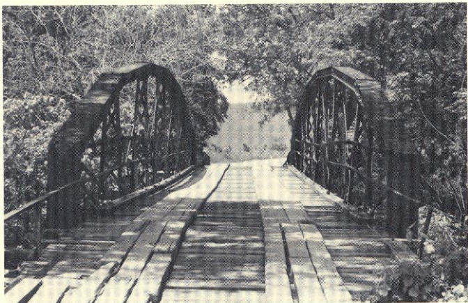
TEXAS LENTICULAR TRUSSES OUTSIDE SAN ANTONIO. All were built in the 1890s by the Berlin Iron Bridge Co. Above left: Yancey Road Bridge over Hondo Creek, Frio County. This is one of the state's two lenticular through-trusses. Above right: County Road 133 Bridge at Dodds Creek, Coryell County, revealing the characteristic double-convex-lens profile created by the top and bottom chords. Below left: County Road 173 Bridge over Plum Creek, Caldwell County. Below right: End panel of County Road 230 Bridge over Plum Creek, Caldwell County. Tex. St. Dept. of Hwys. & Trans. photographs.
