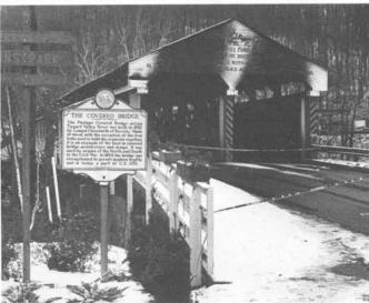
Built in 1852 across Tygart's Valley River in W.Va., the Philippi Covered Bridge is a two-span, 276'long, double-barrel Burr arch truss. It is the work of Lemuel Chenoweth, prolific builder of covered bridges in the state. It is the site of one of the first skirmishes of the Civil War on June 3, 1861. In his *Great American Bridge & Dams* (Preservation Press, 1988), Donald Jackson [SIA] notes that, given the bridge's strategic location, it is remarkable that it survived the Civil War unburned.
