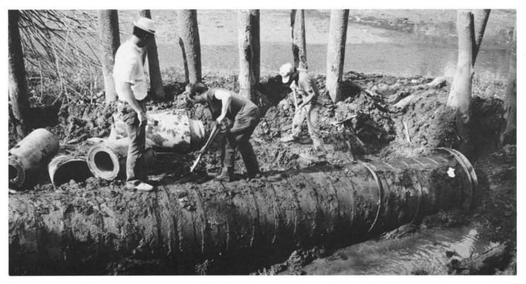
Valentine museum crew (L-R: Lyle Browning, Gregg Kimble, and Greg Galer) removes muck from around the larger of two 1852-53 archimedes screw pumps found in a drained section of the James River & Kanawha Canal, Richmond, Va. Later, the wood-stave pump was lifted out by a Chinook helicopter provided by the U.S. Army Corps of Engineers, whose personnel also had helped dig out the rare 38-ft. artifact. *Photo courtesy of Kathy Franz, Valentine Museum*.
