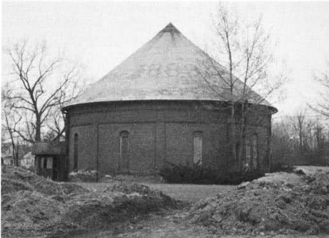
Oberlin's rare 1889 brick gasholder, the only one west of the Alleghenies. It is threatened by a controversial shopping-center project. Photo courtesy of David Perrotta.
