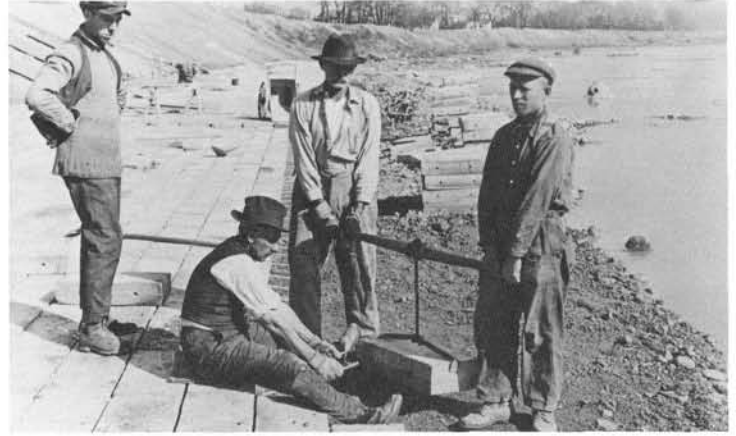
MIAMI, OHIO, CONSERVANCY DISTRICT. Left: Concrete-block manufacturing plant, Dayton, 1919. Right: Building flexible concrete mats, Great Miami River, 1920. Photos courtesy Dept. of Archives & Special Collections, Wright State Univ.
