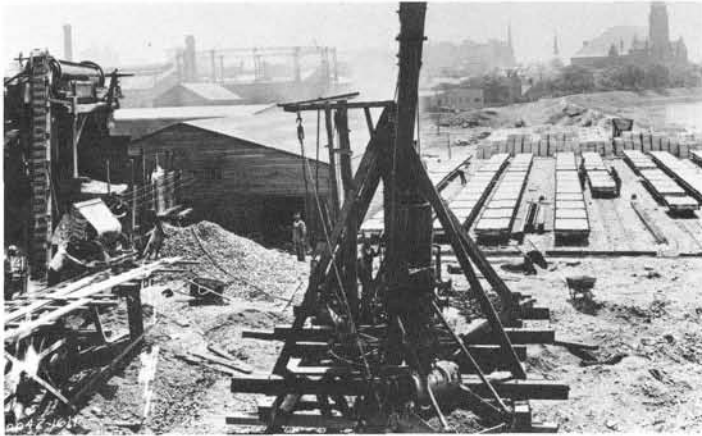
MIAMI, OHIO, CONSERVANCY DISTRICT. Left: Concrete-block manufacturing plant, Dayton, 1919. Right: Building flexible concrete mats, Great Miami River, 1920. Photos courtesy Dept. of Archives & Special Collections, Wright State Univ.
