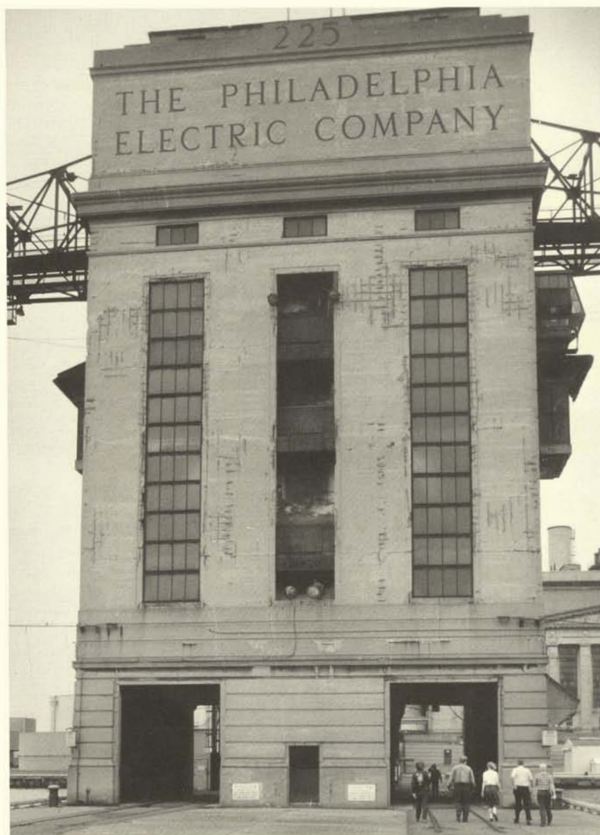
The Richmond Generating Station's coal tower (1925) on Pier 225, Delaware River, for the Phila. Electric Co. Large buckets unloaded barges on both sides; inside, the coal was crushed and sifted, then conveyed to bunkers. R. Frame photo.
