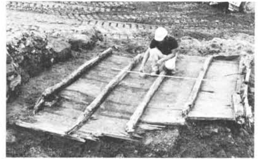
Right. Archeological observer Budd Wilson cleaning section of Morris Canal barge found during demolition of DL&WRR Station in path of highway construction. Remains of canal wall are at the left (6-ft. scale).
