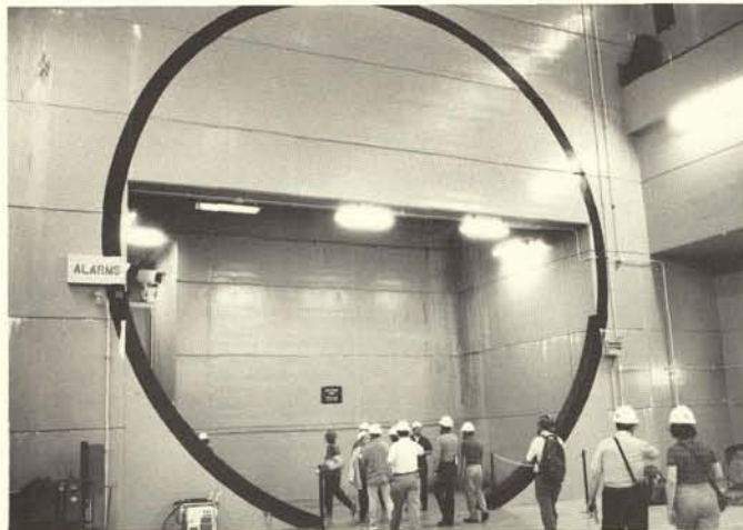
Below: In the Mainstream Station pumphouse, 300 ft. underground, the painted circle shows the scale of the 33-ft.-diam. hardrock tunnel. R. Frame photos.
