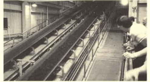
Right: At the end of the process at the Stickney Water Reclamation Plant, sludge ("dewatered wastewater solids") is conveyed [above] to a truck- and rail-loading facility. The Metropolitan Sanitary Dist. locomotive hauls sludge to drying areas in cylinder side-dump DIFCO gondolas [below]. R. Frame photos.
