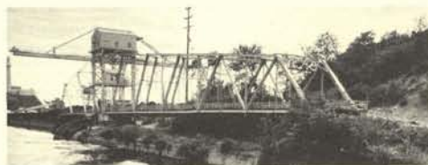
Asymmetrical swing bridge with pivot on shore of Sanitary & Ship Canal. R. Frame photo.
