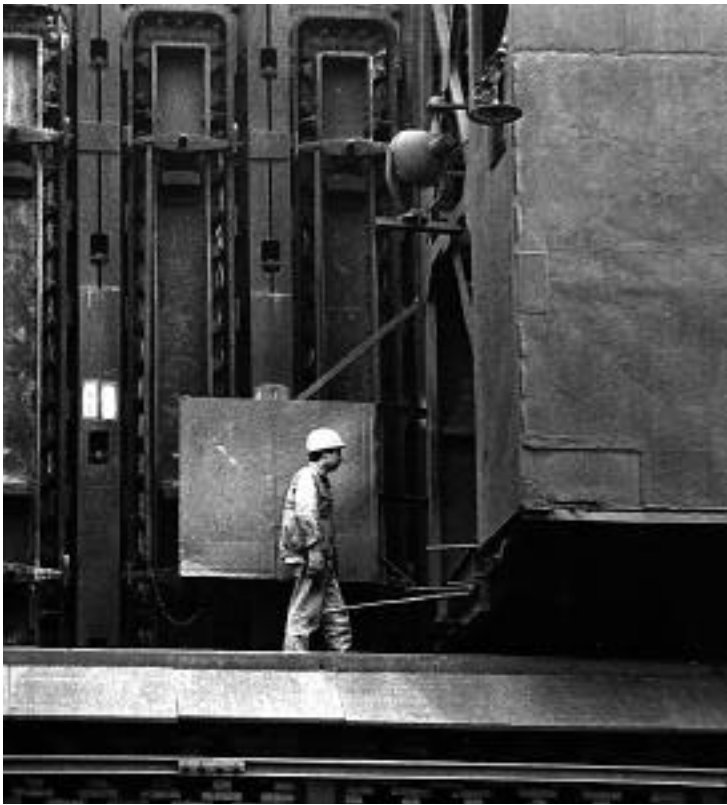
Coke plant, Meishan Iron Works, near Nanjing.
