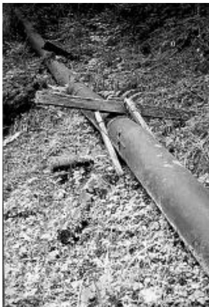
Attached to the headgate was a riveted pipe, which led down to the giant. The view here is looking at the pipe heading up a 50-degree slope.
