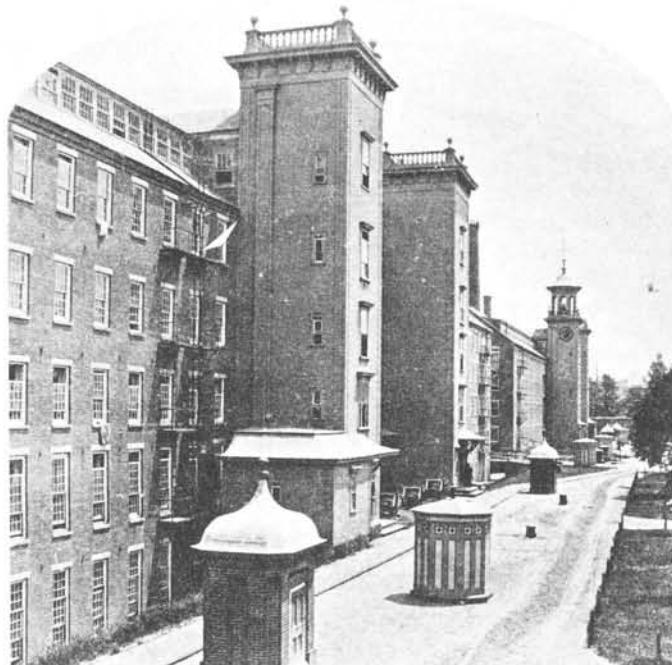
Boott Mill Yard c1880. Not sentry boxes—fire-hose houses. Soc for the Pres of New Engl Antiquities.
