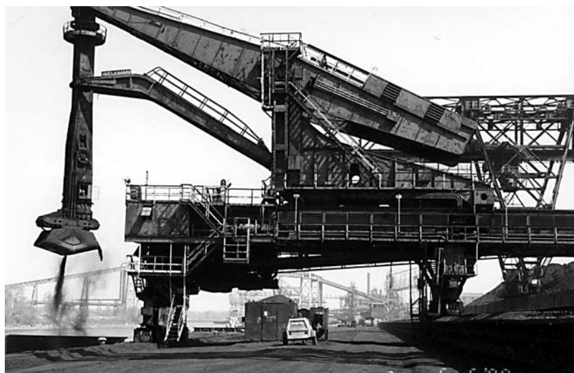
The Hulett unloaders at LTV's South Chicago Works The Hulett's bucket digs coal out of the barge's hold and drops it into a hopper in its framework for transfer to on-site storage. In the late 1890s, the Hulett's greatly improved the efficiency of ore handling, taking over for what was still largely a process of manual unloading.
