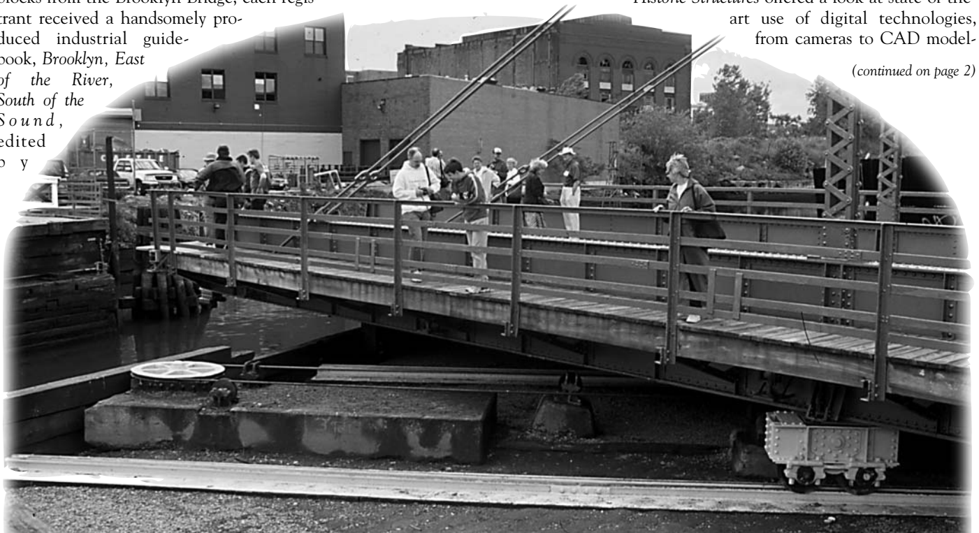
SIAers 'ride' the Carroll St. Bridge, built in 1888-89. The retractile bridge slides horizontally on rails along a diagonal path to clear the channel of the Gowanus Canal.
