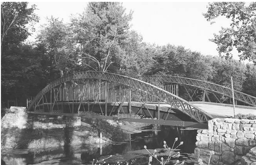
Paint Creek Bridge, built in 1873 by the Massillon Bridge Co.
