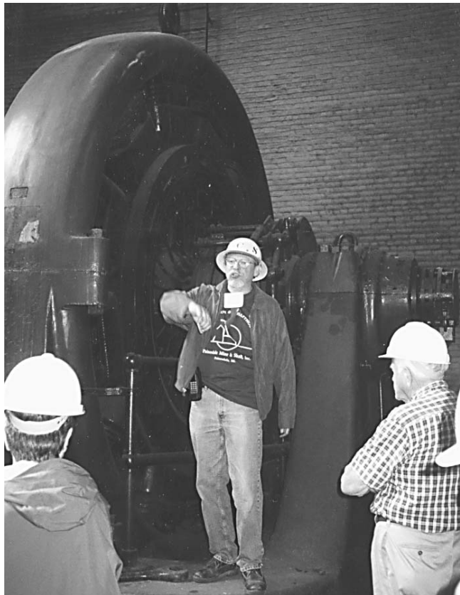
Gerry Weinstein [SIA] explains the operation of the 1,500-kW Westinghouse 'Manhattan' rotary converter at the NCYTA Substation No. 27.
