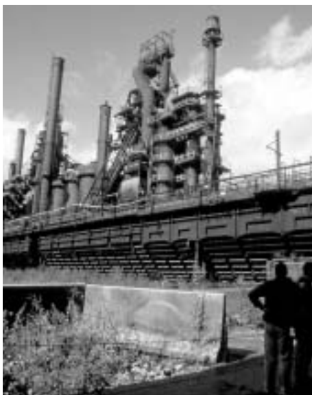
The blast furnaces at Bethlehem Steel. The wide-gauge "Hoover-Mason Line" material-supply railway is in the middle ground.
