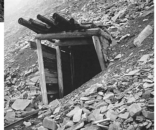
Shaft for waste rock from the Hiorthamma Mine.
