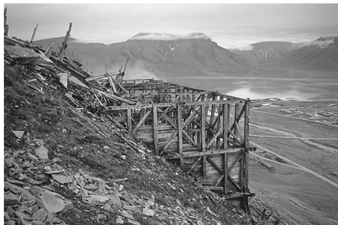
Arctic Coal Co. coal bunker at mine shaft above Longyear Valley.
