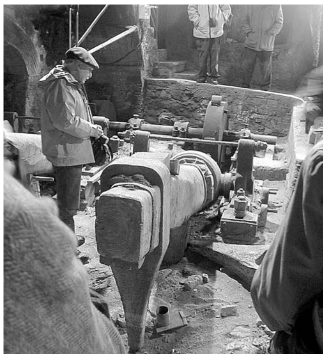
The forge hammer at the Farga Palau in Ripoll.
