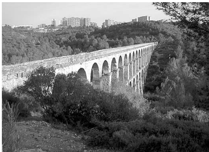
The Pont del Diable Roman aqueduct in Tarragona.
