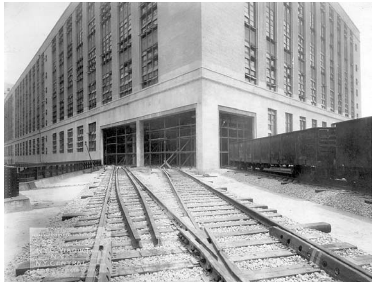
Tracks entering the Morgan Parcel Post Office, which had its own spur bringing trains directly into the building at the second floor level. (The openings are now bricked up.) June 30, 1933.
