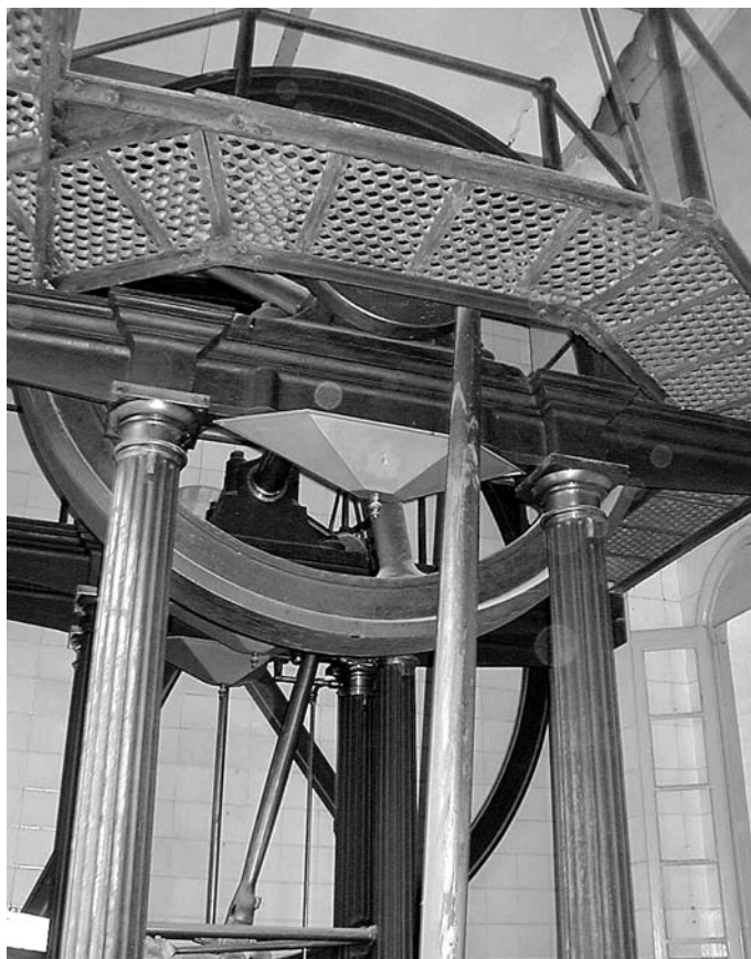
One of the two steam engines at the Montcada pumping station.
