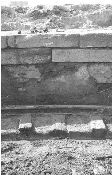
Detail of turntable circumferential bearing rail at base of retaining wall.
