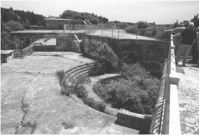
SIA members overlook the disappearing gun platform at Battery Wheaton, Ft. Wetherill, 1907-08.
