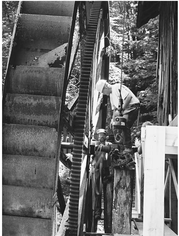
Lou Mogavero of Dearborn, MI (front) and Will Hines of Greeneville, TN, prepare for the crane to lift the waterwheel just enough to slip a temporary support in place.
