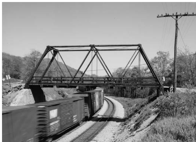
The Warren through-truss, cast- and wrought-iron bridge at Meyersdale, PA, was built in 1871 by the B&O RR to a design of engineer Wendel Bollman. The bridge will be relocated to a nearby rails-to-trails pathway.
