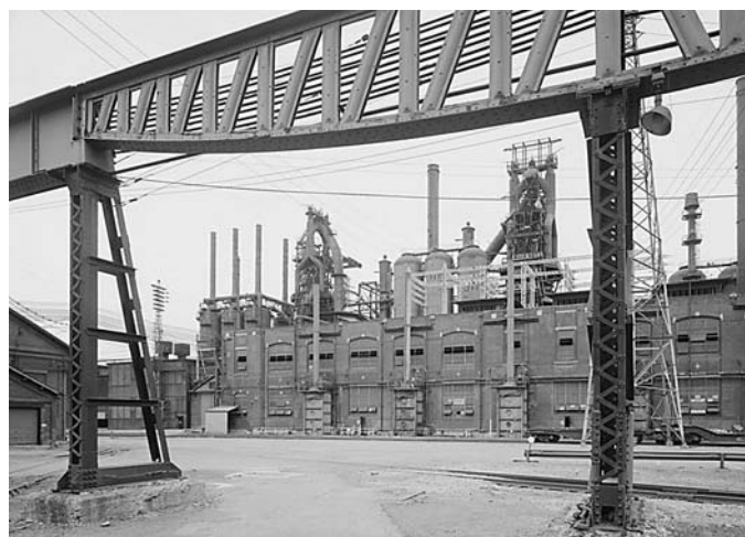
General view of Bethlehem Steel’s blast-furnace plant in Bethlehem, 1988. Furnace A, built in 1908, to the left; in the foreground is the turbo-blower and blast furnace gas-powered electric generating station, built in 1919. HAER PA-48-1.
