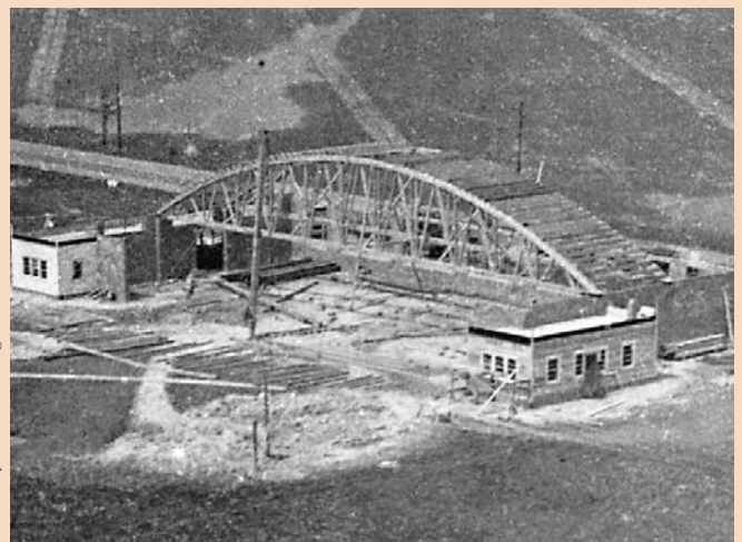
A c. 1935 construction photo shows the timber roof trusses of the Bellanca Hangar.
