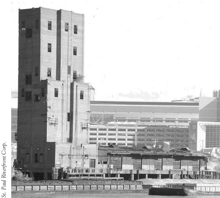
The St. Paul Municipal Grain Terminal from across the Mississippi River, with downtown St. Paul in the background. The transfer elevator is the tall reinforced-concrete building (left). The sackhouse or flathouse is the one-story, brick structure extending to the right, with its five large overhead doors opening onto the dock. In front of the buildings are several large barges.
