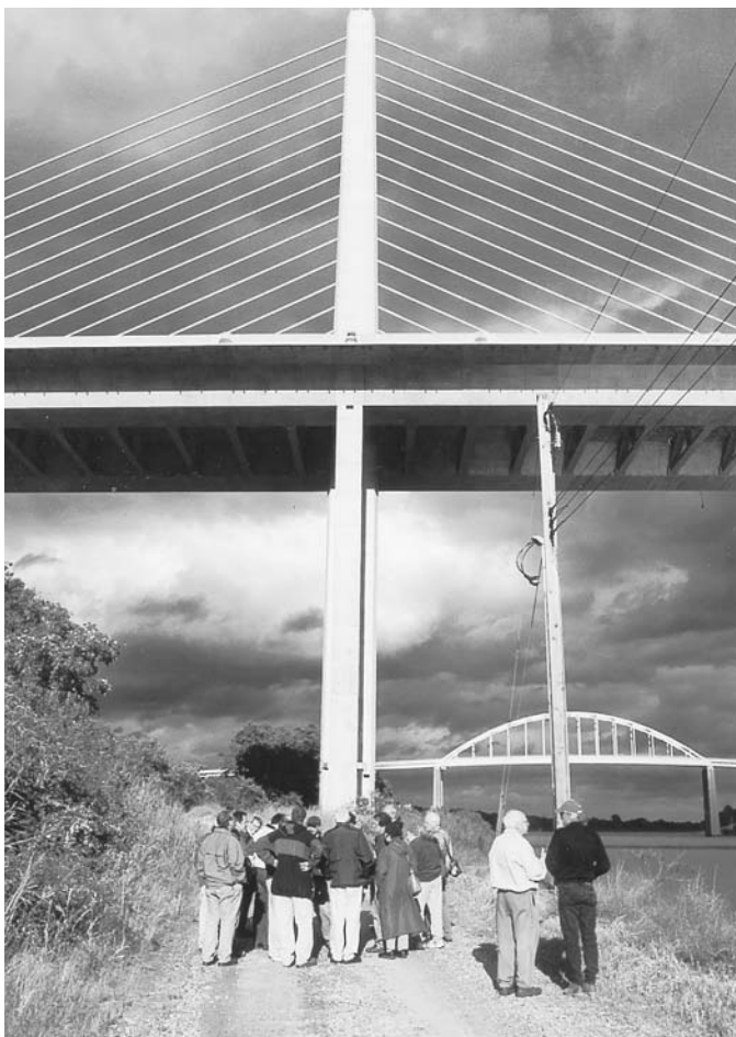
Bridge tour participants contemplate the Delaware Route 1 bridge over the Chesapeake & Delaware Canal (a cable-stay bridge completed in 1995). The St. Georges Bridge, a tied-arch built in 1940-42, is in the background.
