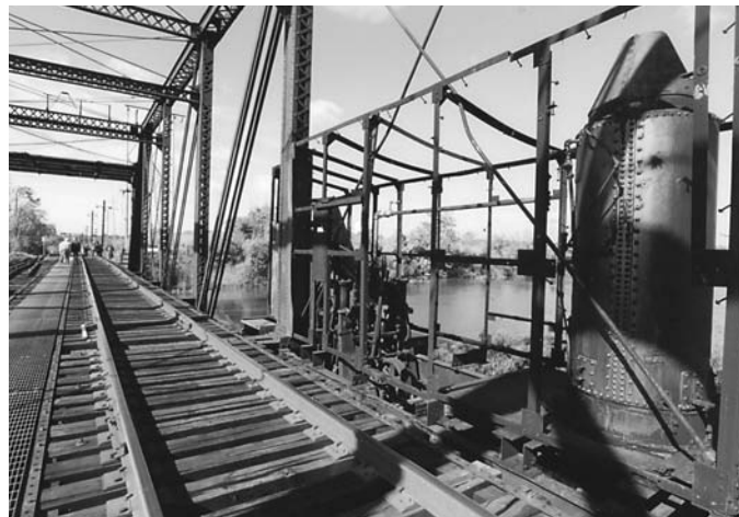
The non-operating stationary steam engine and boiler operating system (right) on the Pennsylvania RR's swing-span bridge (c. 1888) over the Christina River.
