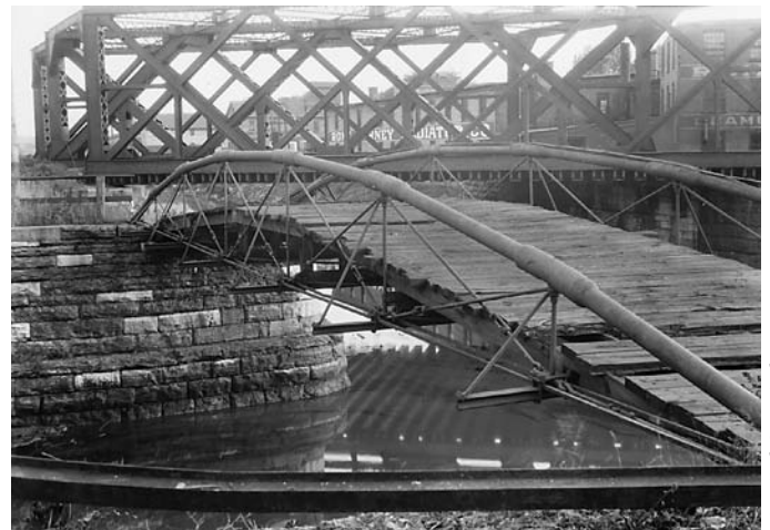
Whipple's Pipe Arch Bridge, at Rome, NY; undated photograph.
