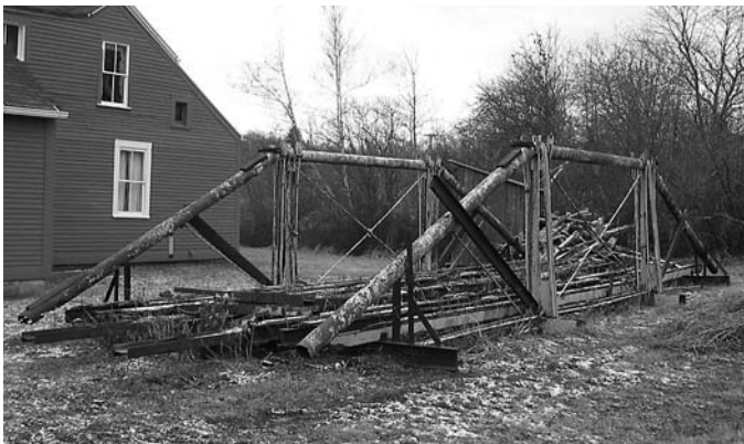
Holiday Road (Dalton) Ball Pipe-Truss Bridge in storage at the Windsor (MA) Historical Museum. The bridge is being disassembled, rehabilitated, and re-erected as a pedestrian bridge at the University of MA—Amherst.
