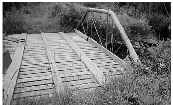
The Windsor Bush Road Ball Pipe-Truss Bridge is abandoned and threatened with loss.
