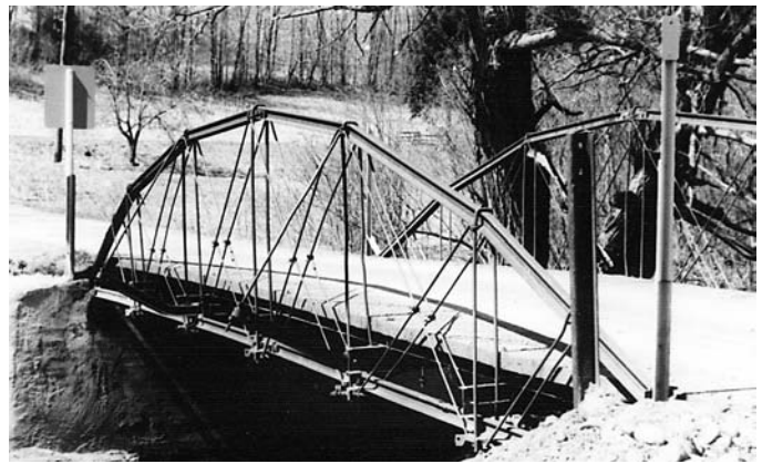
Patented Railroad Iron Bowstring Truss Bridge, Nubia, NY, built c. 1877 by the Groton Iron Bridge Co.
