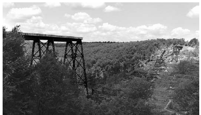
Two days later, eleven of the viaduct's 20 towers lay twisted on the valley floor.
