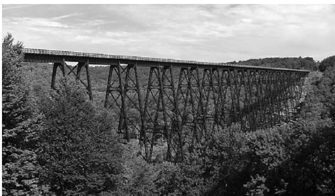
The last known photo taken of the Kinzua Viaduct prior to the tornado on July 19, 2003.
