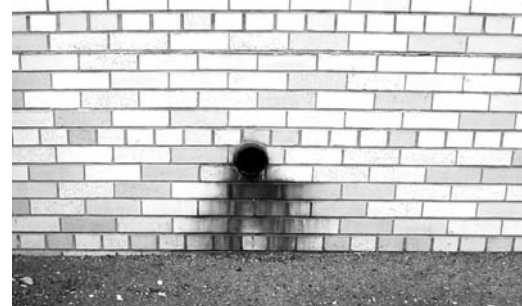
Floor drain outfall corresponding to sectional drawing.
