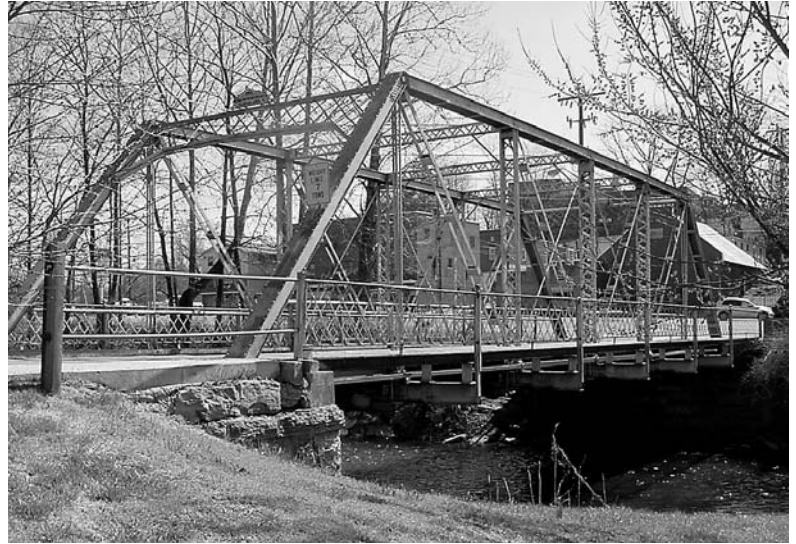
Happy's Bridge, Marion, Virginia. Fabricated by the King Iron Bridge Co. in 1885.
