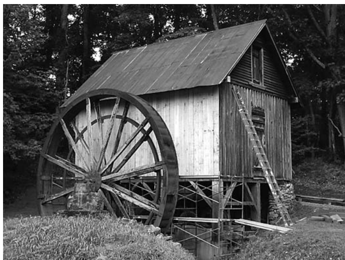
The c. 1887 Francis Mill after the completion of the 2005 workshop, showing the new siding on the east side and new top plate beam.
