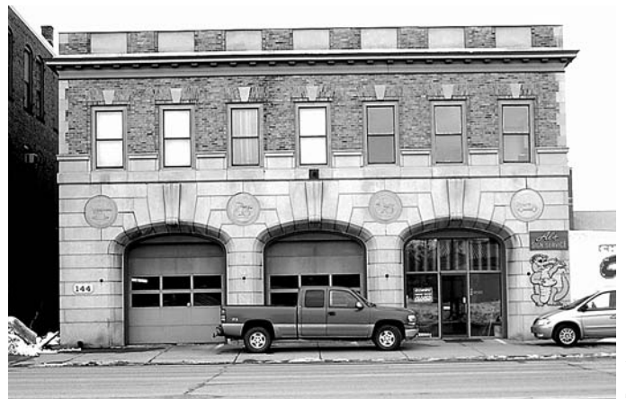
Erie City Fire-station (1931), once a symbol of civic pride, is now little appreciated.
