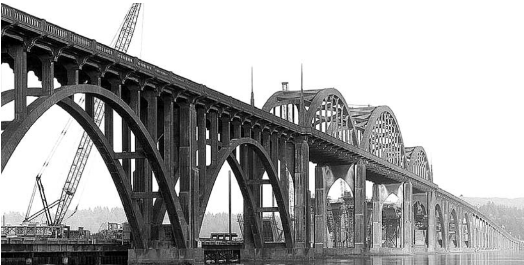
The loss of the magnificent Alsea Bay Bridge in the early 1990s was a wake-up call to Oregonians that their historic bridge legacy was in jeopardy. The reinforced-concrete tied thru-arch bridge at Waldport was designed by engineer Conde B. McCullough and opened in 1936. HAER OR-14.
