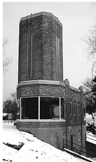
Pettibone Creek Hydroelectric Station, built in 1939, restored in 2006. Design by Albert Kahn.
