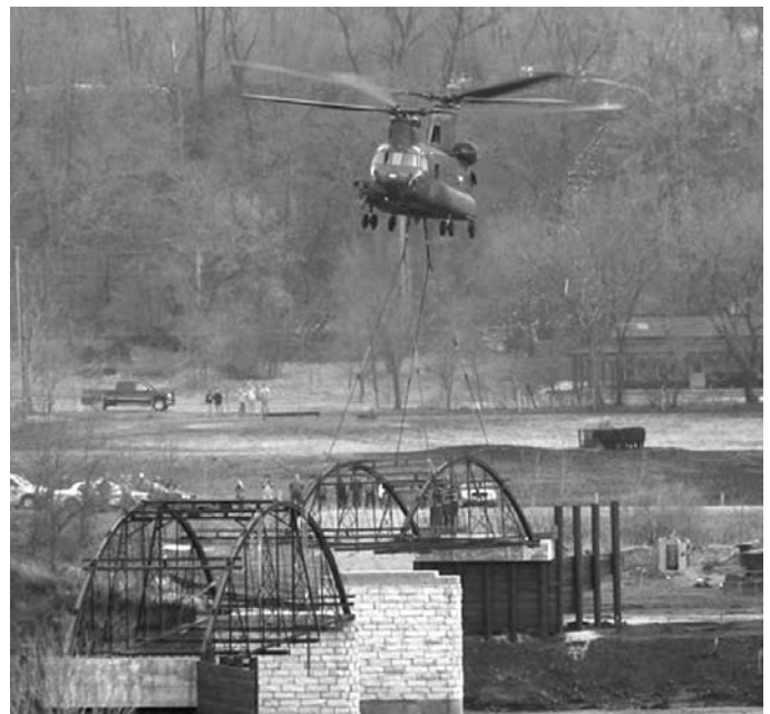
A Chinook helicopter places the Hale Bridge's center span on its new stone-faced concrete piers in Wapsipinnicon State Park.
