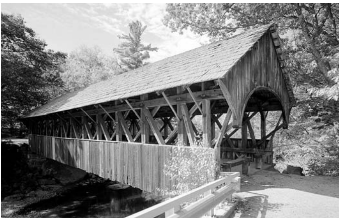
Sunday River Bridge, an 1872 Paddleford truss in Maine, is also known as Artist's Bridge because it has become a popular artistic subject.
