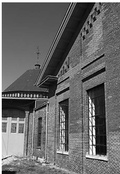
Restored brickwork at the Martinsburg Shops.
