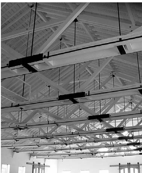
Restored roof trusses of the Bridge & Machine Shop.
