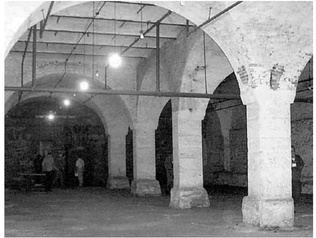
Beer storage and lagering cavern, Lemp Brewery
