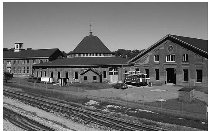
A recent view of the B&O RR's Martinsburg Shop complex shows the extensive rehabilitation work.
