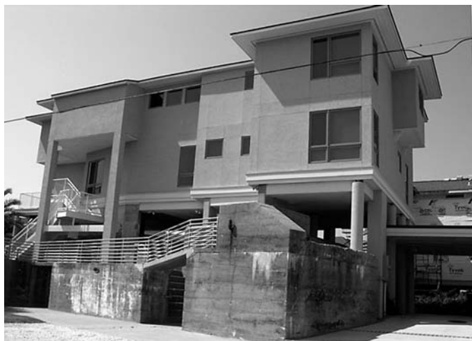
Modern beachfront housing uses a rapid-firing gun battery for a secure foundation.
