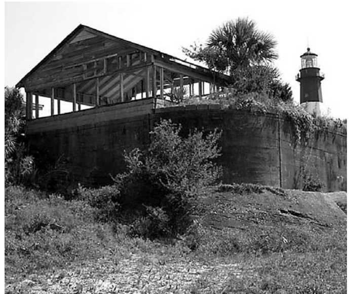
A battery that was built for 12-in. mortars now supports vegetation and the frame for an abandoned house, with Tybee Island Lighthouse in the background.
