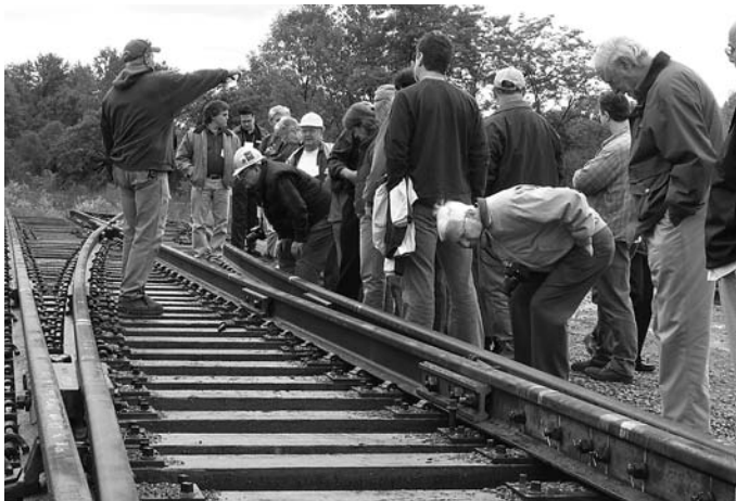
At L. B. Foster Co., a worker explains pre-fabricating a switch. The pieces will be match-marked, disassembled, and then shipped to a railroad in Alabama.
