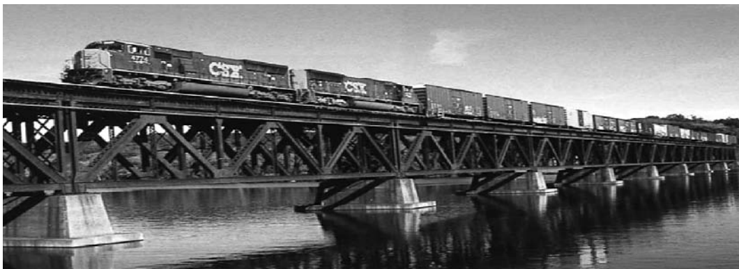
The current Mechanicville crossing. Three parallel Warren trusses support each span.
