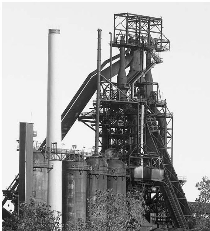
The blast furnace at WCI Steel (former Republic Steel) in Warren, OH.
