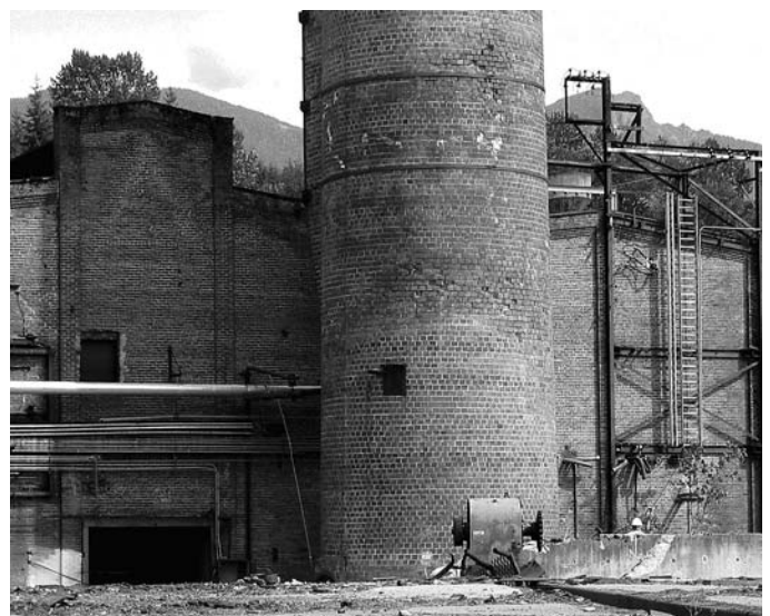
West façade of the powerhouse and brick stack, 2006.
