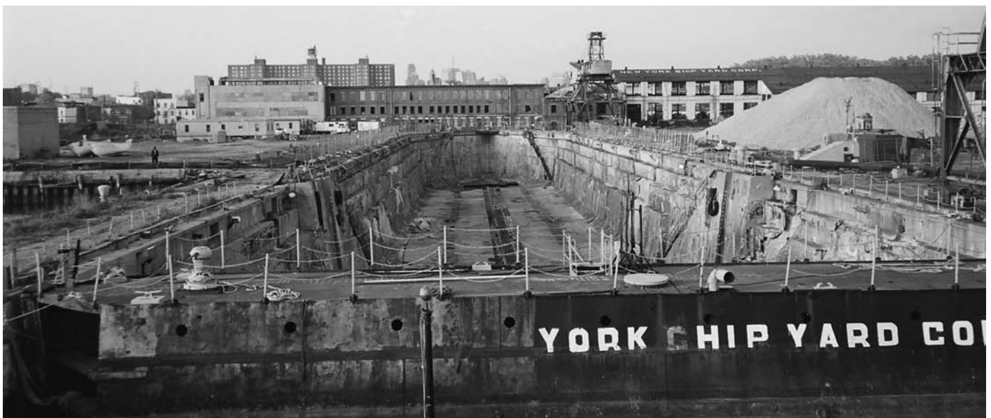
Graving Dock No. 1 (May 17, 2006). The pumphouse is behind the gantry crane. In the foreground, the caisson has lost the "New" in "New York Shipyard Corporation."
