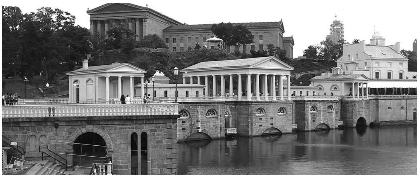
Fairmount Water Works has been beautifully restored as an interpretive center and was the site for the 2007 conference's banquet.
