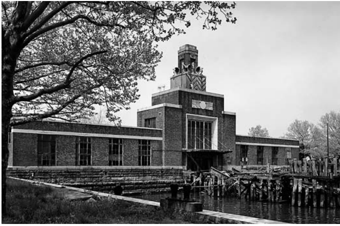
Ellis Island Ferry Terminal, prior to restoration.
