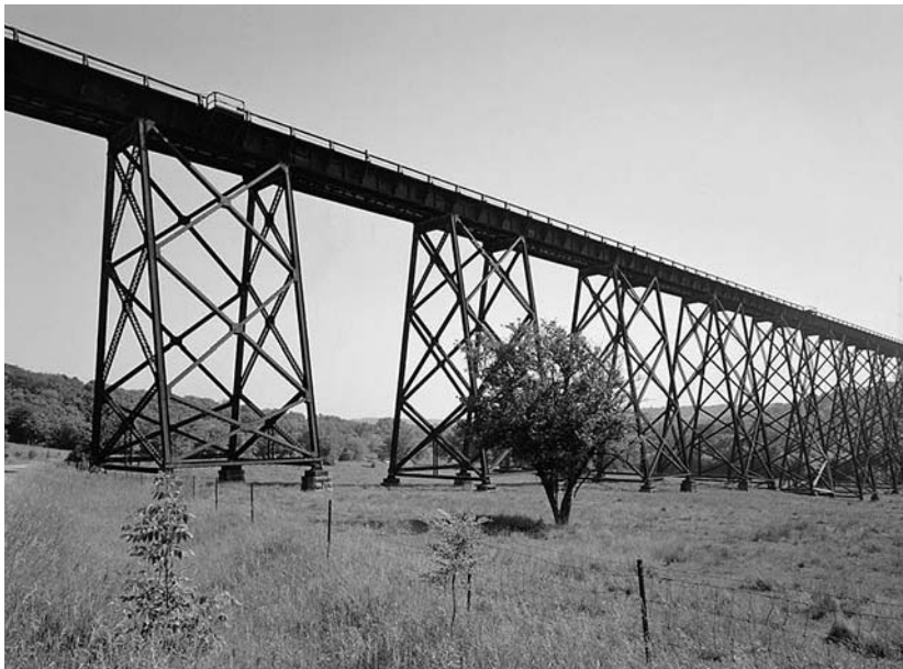
Kate Shelly Bridge near Boone, Iowa.
