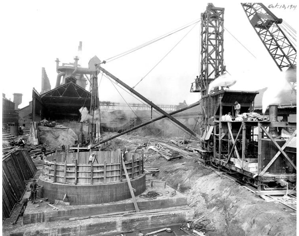
Corrigan McKinney Steel, 1914. Construction of Blast Furnace #3 with older style furnace in the background.
