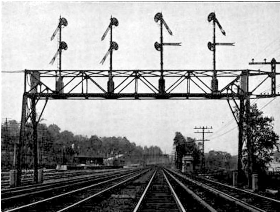
Four-track signal bridge showing lower-quadrant semaphore signals, NY Central & Hudson River RR (The Railroad Signal Dictionary, 1908, p. 102)
