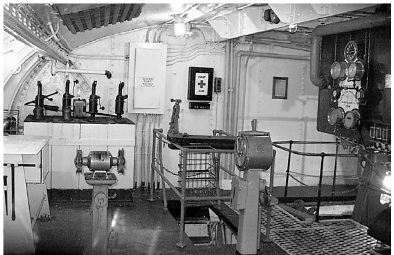
The upper level of the engine room.
