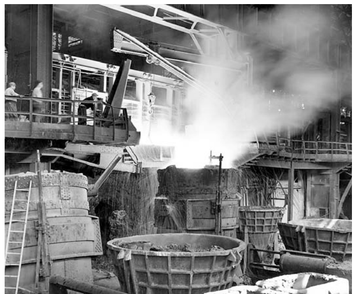
Otis Steel, ca. 1935. Tapping the open hearth.
