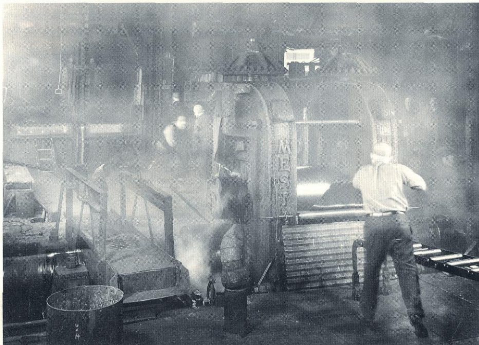
Republic Steel's Warren Works, ca. 1930. Hand-rolling silicon-steel sheets.
