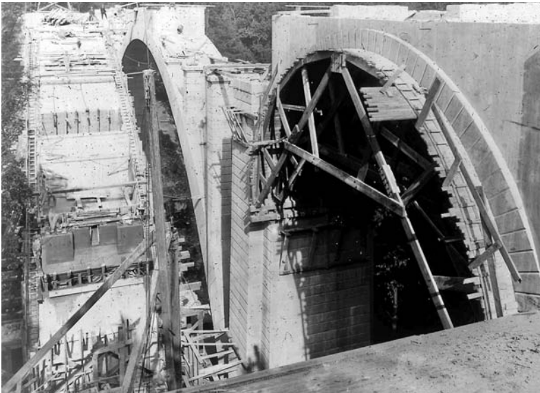
Arch ribs in various stages of completion.
