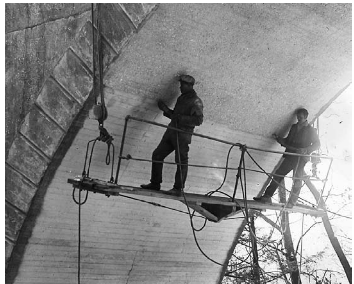
Workers finishing the intrados of the arch.
