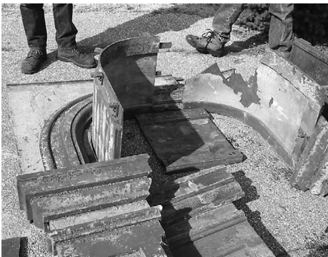
Pieces of the firehouse façade. Most retain their original tabs for attachment to each other.
