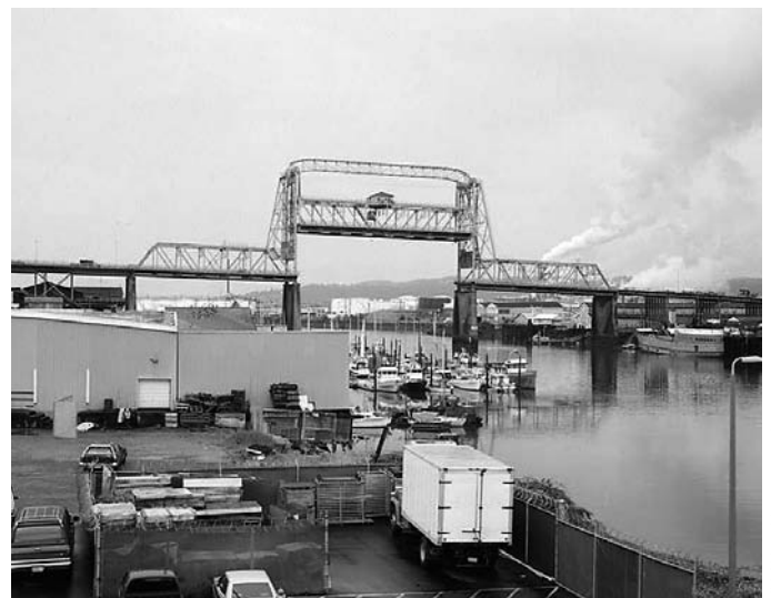
The Murray Morgan Bridge in the open position.
