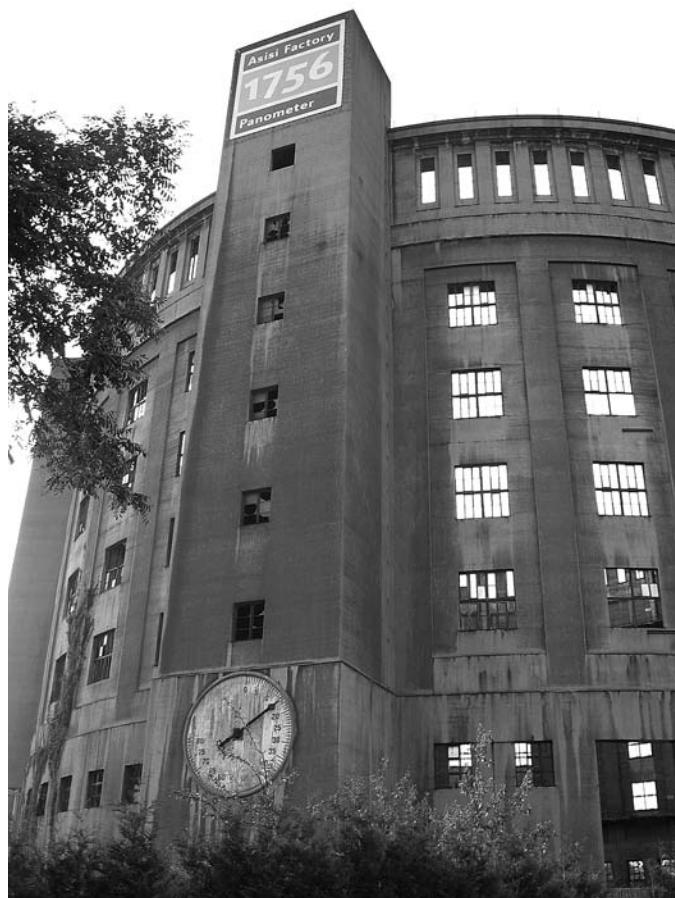
In 1907-08, Dresden's Erlwein gasometer house was built in reinforced concrete.
