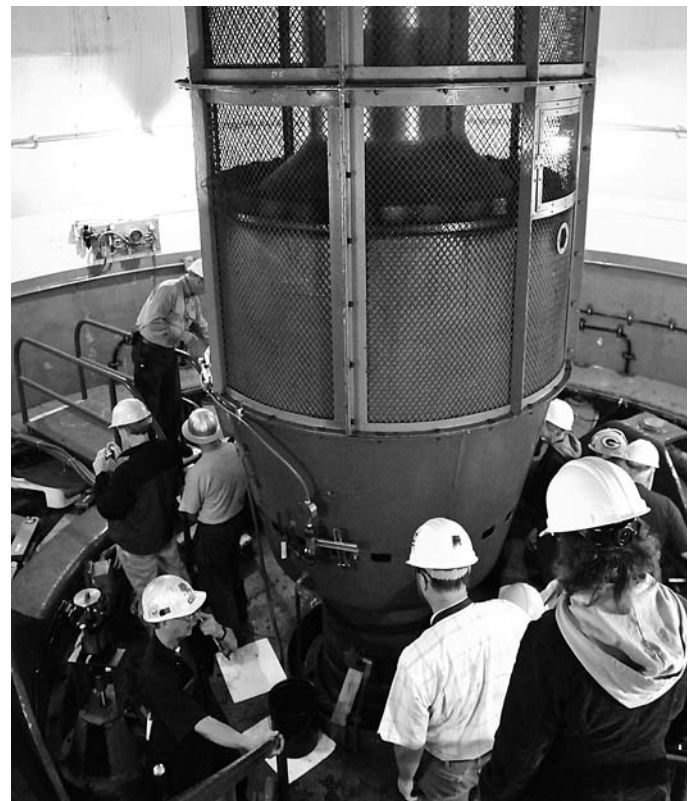
In the turbine pit at the TVA’s Chickamauga Dam.
