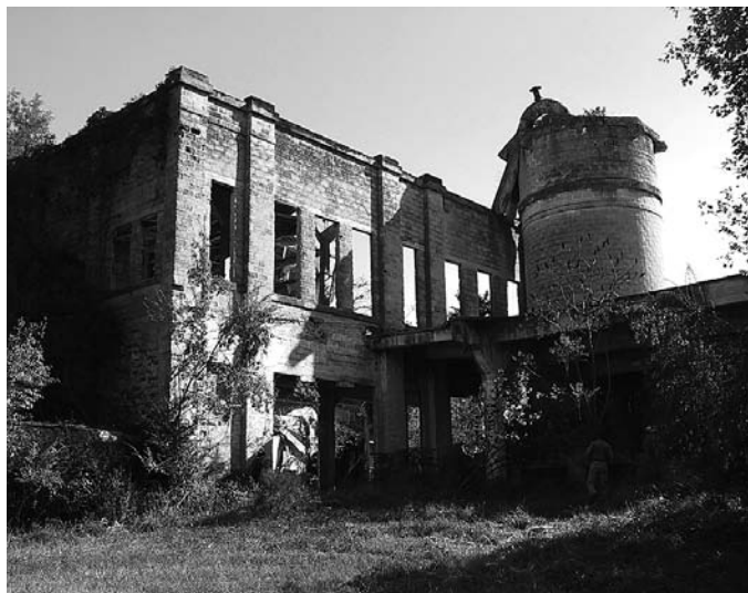
Ruins of the Gager Limestone Manufacturing Co.
