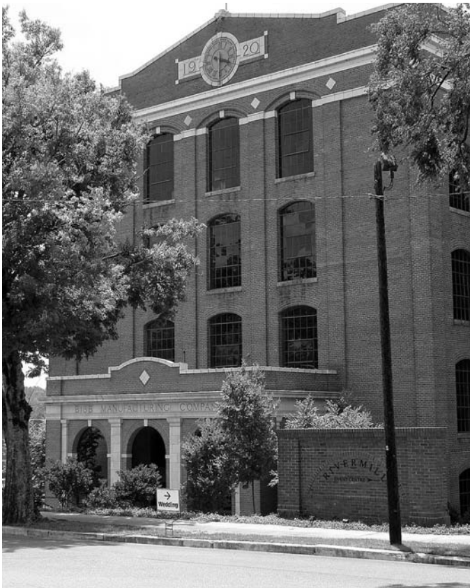
Columbus's Bibb Mill was destroyed by fire.
